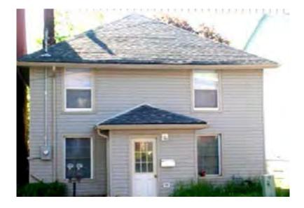
The 163 Bagot Street building is clad in modern materials of no heritage significance. The location and footprint of the building suggest that an older 2-storey wood dwelling could exist underneath the exterior of the present structure. That building was erected between 1856 and 1865. By 1924 it was clad in brick.
