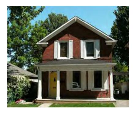
The 129 Bagot Street building is a 2-storey brick house with simple ornamentation and rectilinear features. The building has short decorative pendant at the apex of its front gable roof. The roof has return eaves, and a strong overhang with a series of small dentils. The cornice and entablature are otherwise plain. The structure's large plain windows, and flanking shutters, are of no heritage value. The first-storey façade features a full-width open balcony with plain wood pillars.
