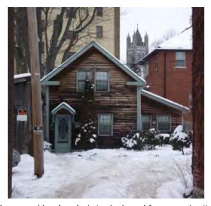
what would have, by then, been considered modest standard wood-frame construction was utilized. The building was originally rough cast likely as fire protection for a residence so close to the bakery and this has been removed in recent years. The current shiplap siding may have originally been the sheathing for the furred out stucco but confirmation would require closer examination. It is the only frame dwelling on the Block.
